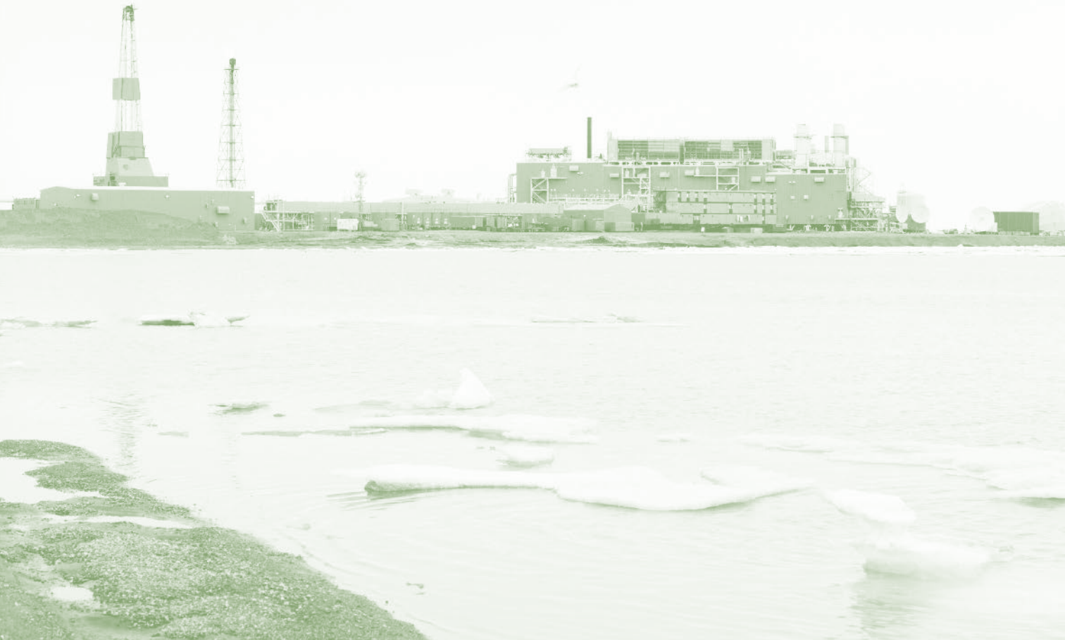
An oil drilling rig and a production facility in Prudhoe Bay, Alaska. Conserving Alaska's public lands became especially controversial during the 1970s as the OPEC oil embargo led to increased gas prices and inflation, which in turn led to an expansion of federal lands for domestic oil and gas production. Concurrently, President Jimmy Carter used the Antiquities Act to designate more than a dozen national monuments in Alaska, withdrawing them from development. The debate over Alaskan oil production continues to this day. HABS AK,15-PRUBA.V,1, Library of Congress
